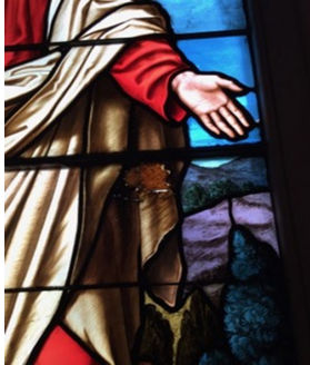
Before—one of the panes removed for repair
